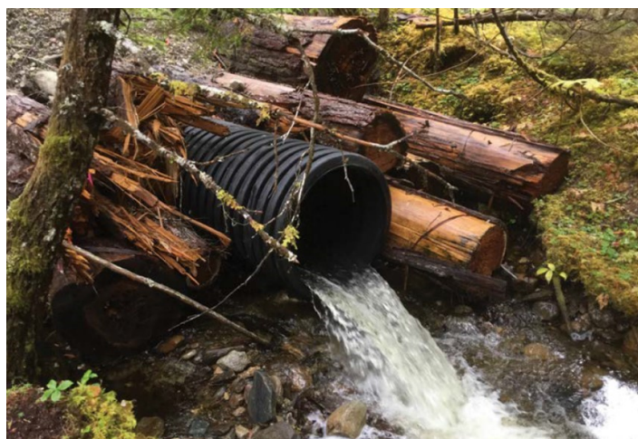
Temporary structure over creek crossing.
