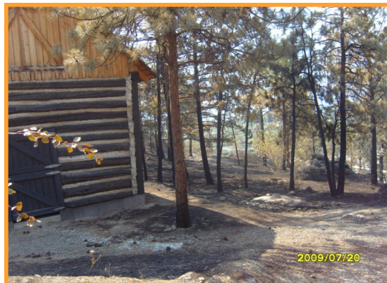
These photos were taken after the Glen Rosa fire in Kelowna, BC. Fuels had been reduced in the areas adjacent to the structure, the fire reached the structure but caused little damage.
